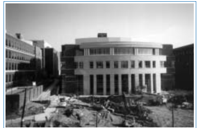
Crews apply the finishing touches to the face of the library.
