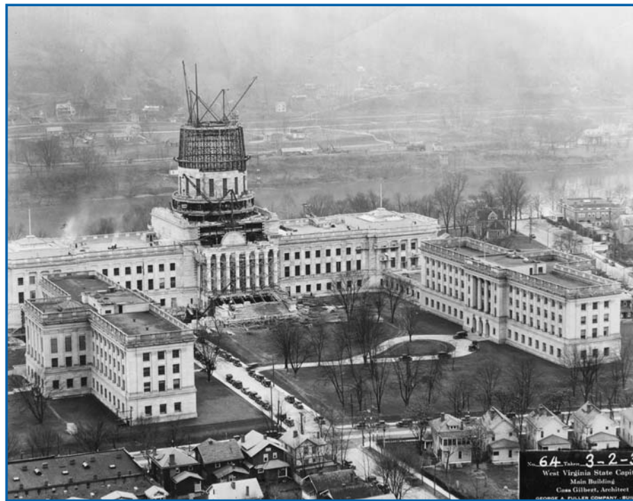
The State Capitol under construction, circa 1931.
